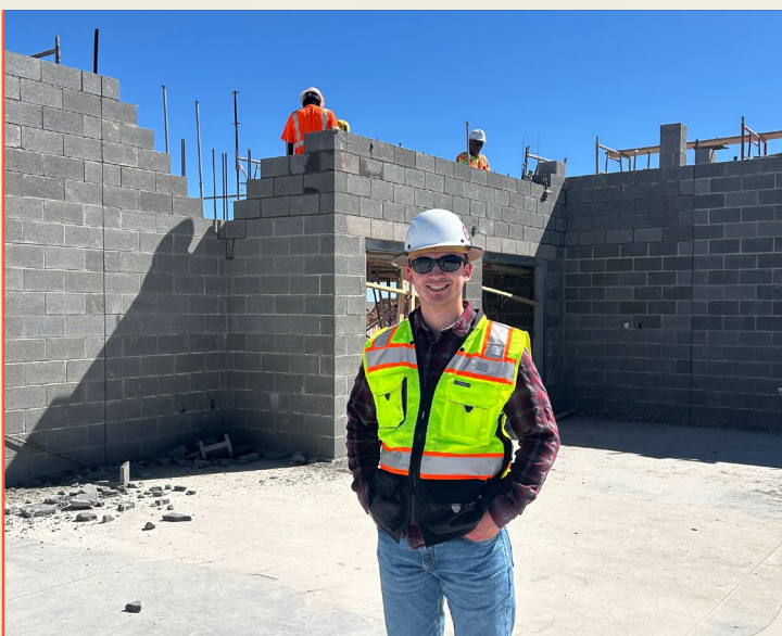
Sealaska Shareholder and previous intern Jay Brendible, working on site as a Project Engineer for Sealaska Constructors.
